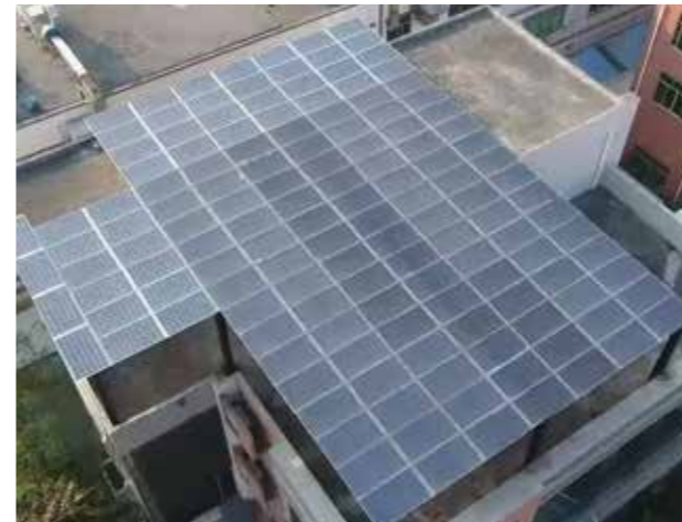
Li Hua Ltd. - Dongguan, China Capacity : 34 kW Annual output : 37,400 kW/h Annual income : RMB 526,360
