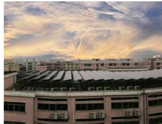
ProVista Group - Dongguan, China Capacity : 350 kW Annual output : 392,000 kW/h Annual income : RMB 509,600
