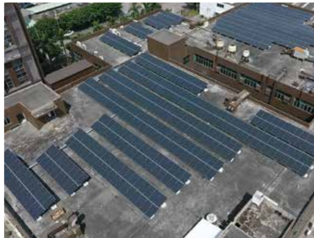
G.E.W Electric Ltd. - Dongguan, China Capacity : 200 kW Annual output : 20,000 kW/h Annual income : RMB 326,600
