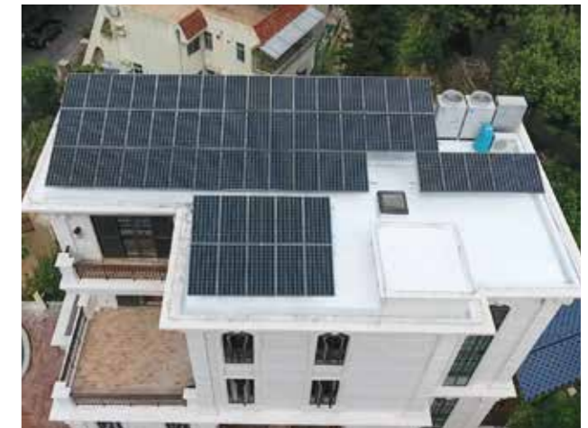
Changan Diamond Villa - Dongguan, China Capacity : 12 kW Annual output : 13,440 kW/h Annual income : RMB 18,412
