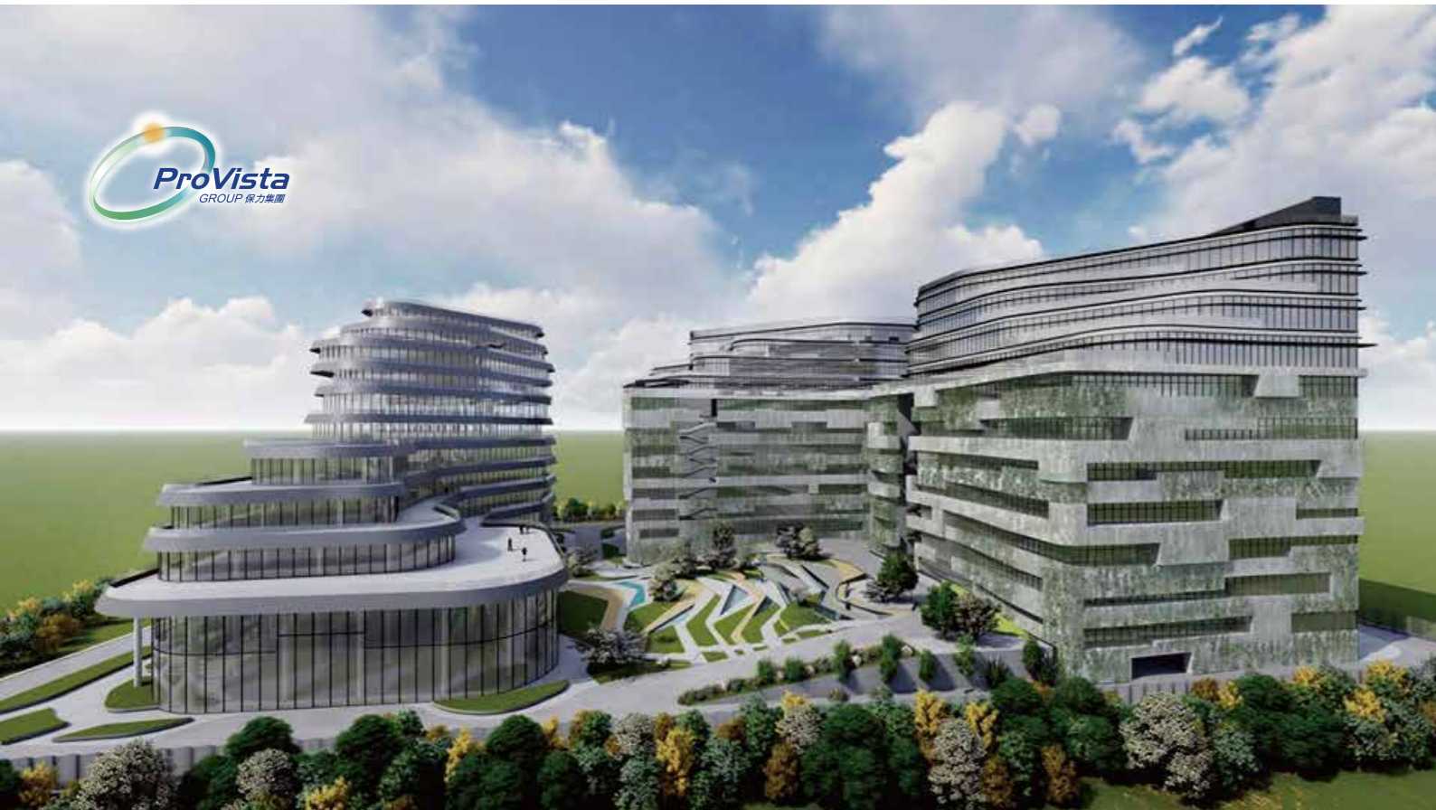
ProVista Inno Park will become the first international innovation technology & creative industry park in Dongguan Songshan Lake
