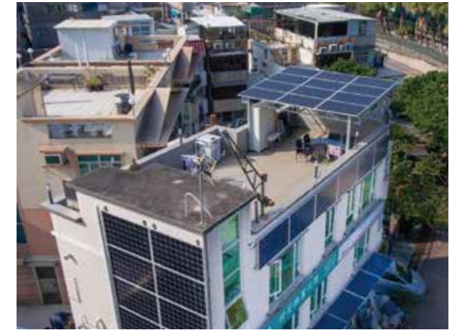
Pan Chung - Taipo, Hong Kong Installed Capacity : 3.6 kW/6.3 kW Annual output : 16,560 kW/h Annual income : RMB 59,400
