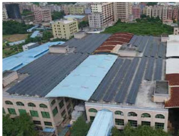
Sinomax Furniture Ltd. - Dongguan, China Capacity : 1,157 kW Annual output : 1,272,000 kW/h Annual income : RMB 2,587,200
